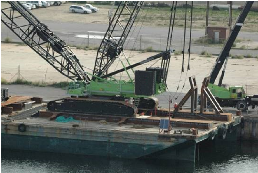
Photo showing an example of load spreading
